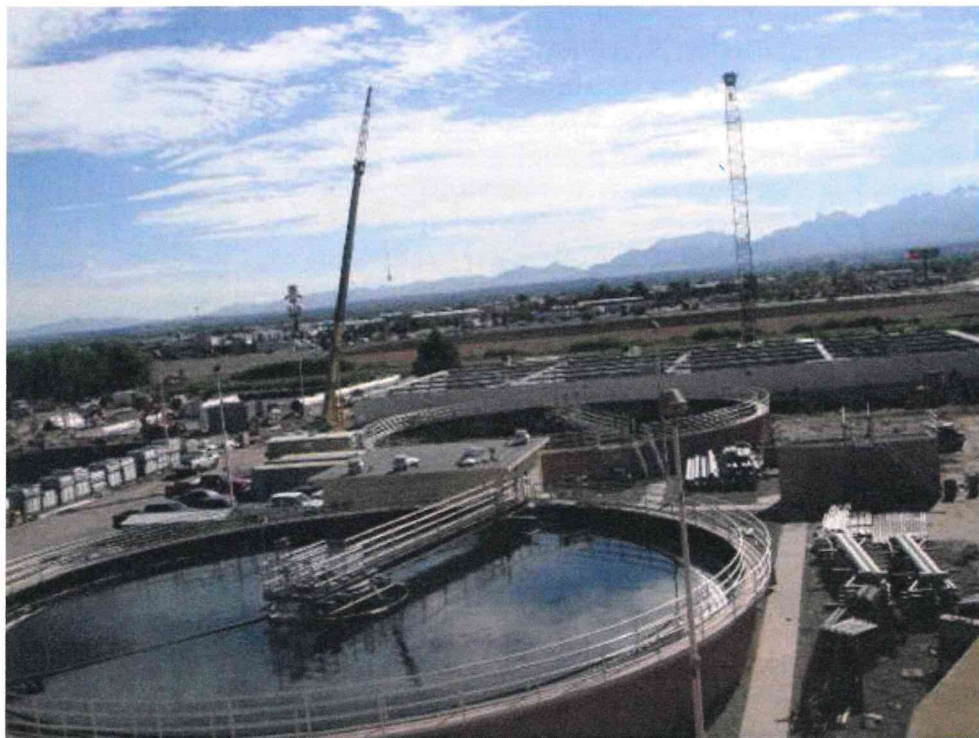
The primary clarifier (foreground) at the Las Cruces Wastewater Treatment Plant was one of several places where wastewater samples were taken for the study.
